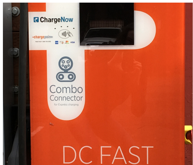
This fast charger in Dunsmuir, CA, has an SAE Combo connector, so it is only compatible with American and European car models. Credit: Staff.
