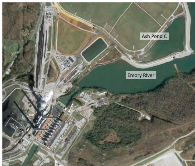
At the Kingston Fossil Plant, Ash Pond C contained decades worth of toxic coal ash waste. When the coal ash pond's dike failed, more than 1 billion gallons of coal ash waste flowed into the nearby Emory and Clinch rivers. 12 Image: U.S. EPA
