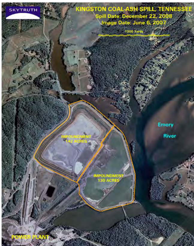
Often, coal ash ponds are separated from water by only a thin retaining wall, as was the case for a pond at the Kingston Fossil Plant in Tennessee, the site of one major spill. Credit: Skytruth via Flickr (CC BY-NC-SA 2.0)
