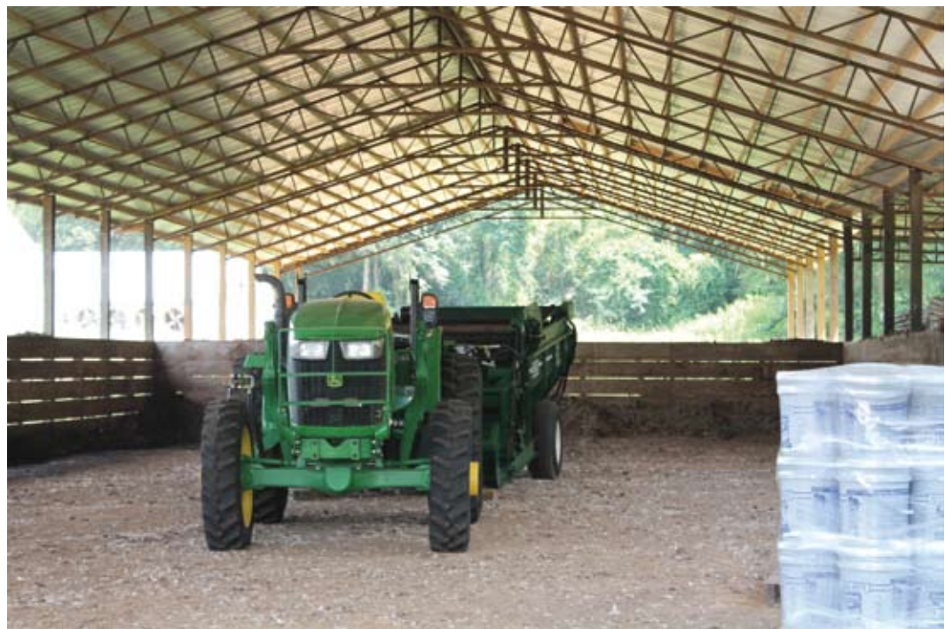
Construction of this poultry litter storage facility in Hazlehurst, Mississippi, was funded by the USDA’s Environmental Quality Incentives Program. Photo: Judi Craddock, USDA NRCS via Flickr, CC BY 2.0.
